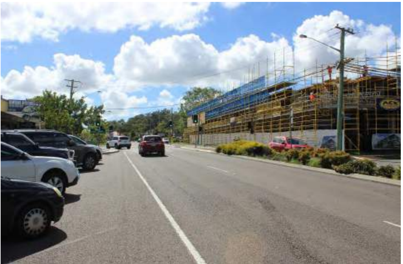
Photograph 12 – Signalised pedestrian facilities adjacent to the site in King Street.
