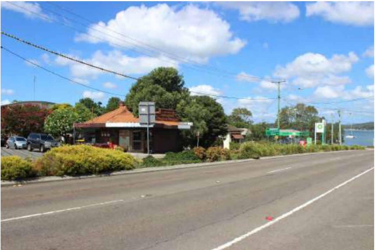
Photograph 1 - Existing Site Development – King Street
