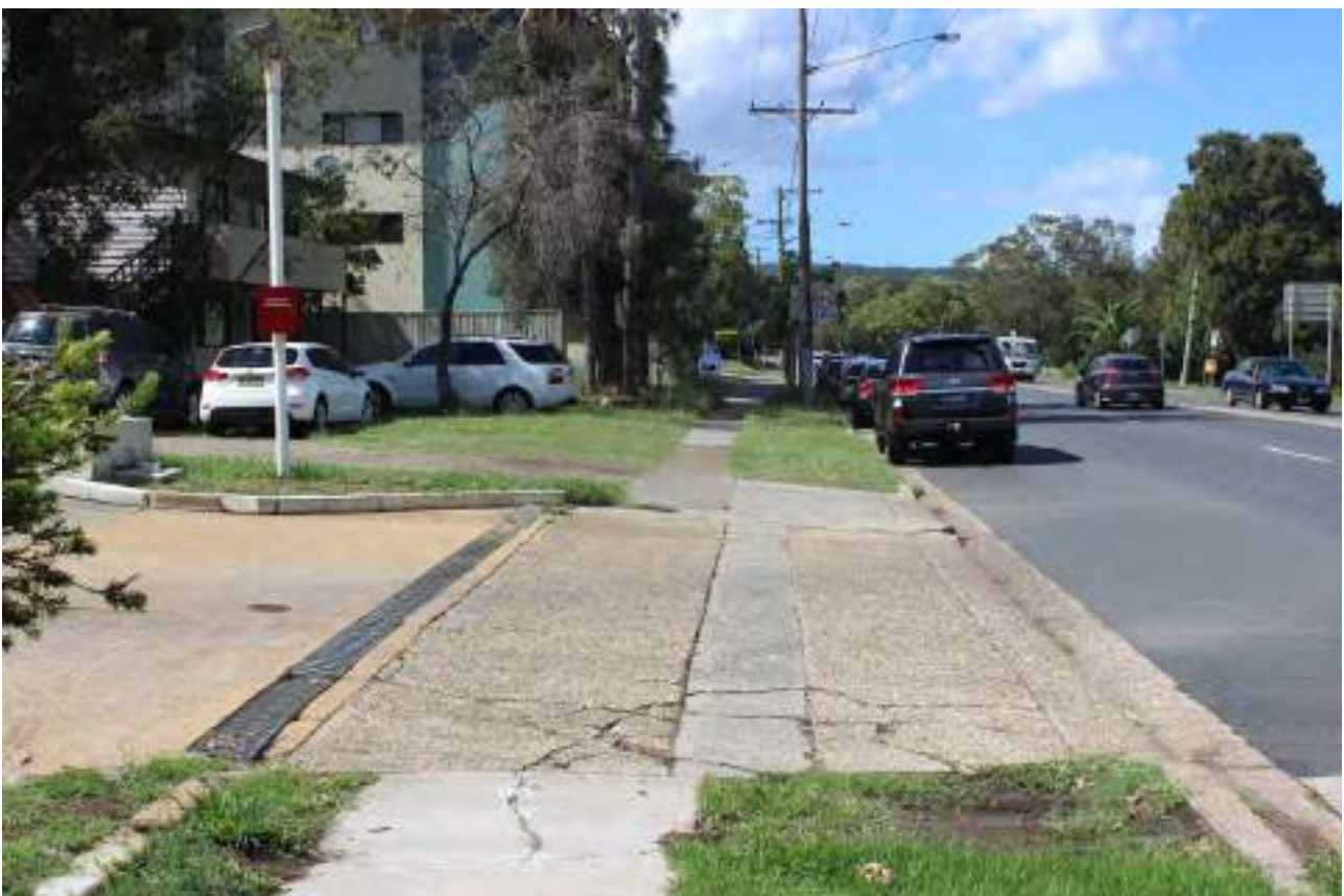
Photograph 4 - Existing Vehicular accesses – The Esplanade
