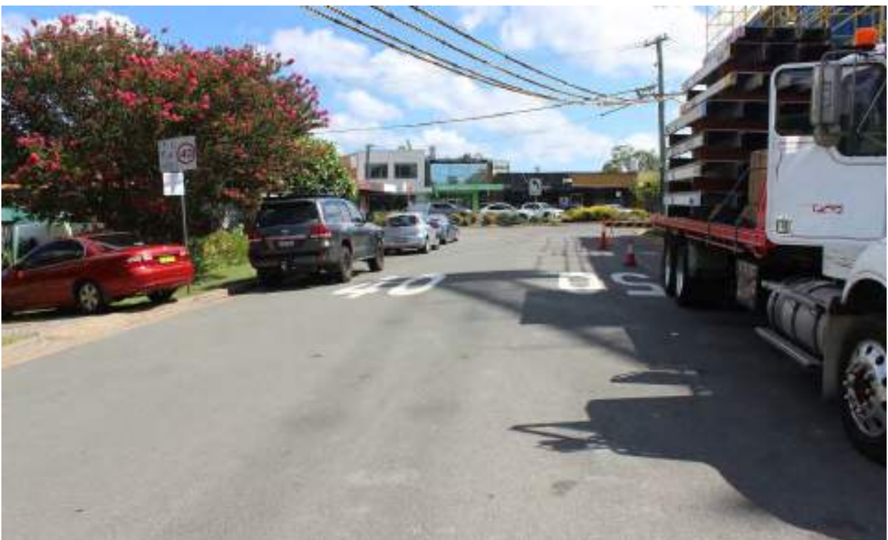
Photograph 7 – Howard Street near the site
